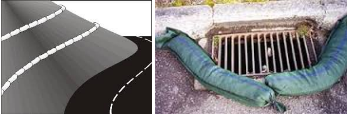
Figure 8-4: Example of sand bag use
