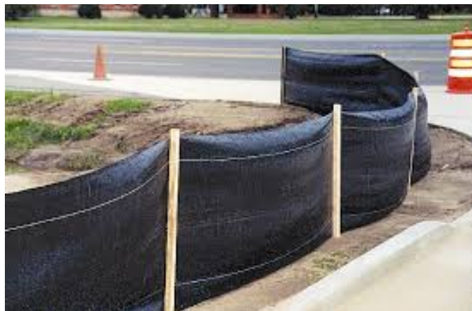
Figure 8-3: Example of silt fence
