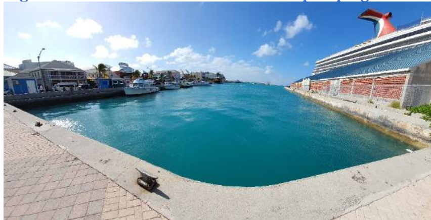
Figure F-2: Reclamation area view from pumping location
