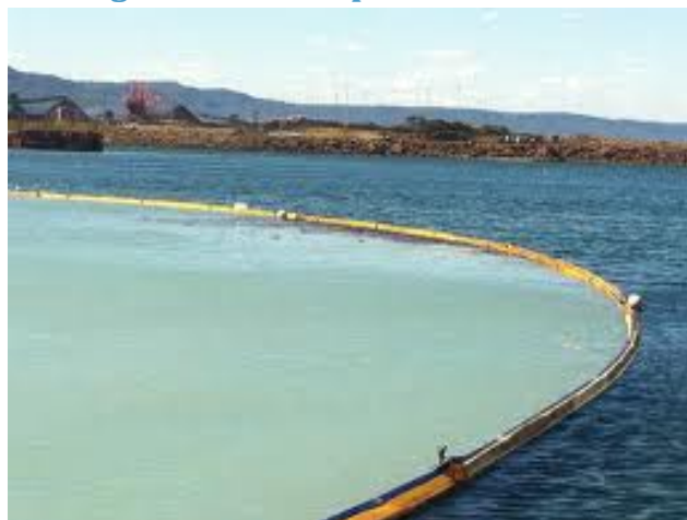
Figure 8-5: Example of silt curtain
