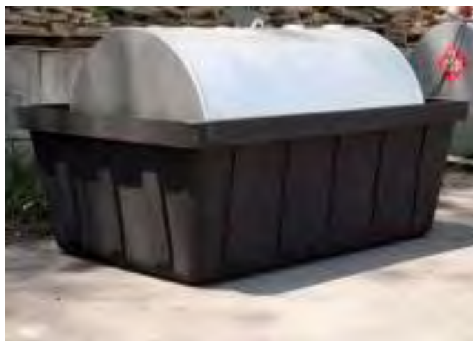
Figure 4: Fuel tank storage containment system
