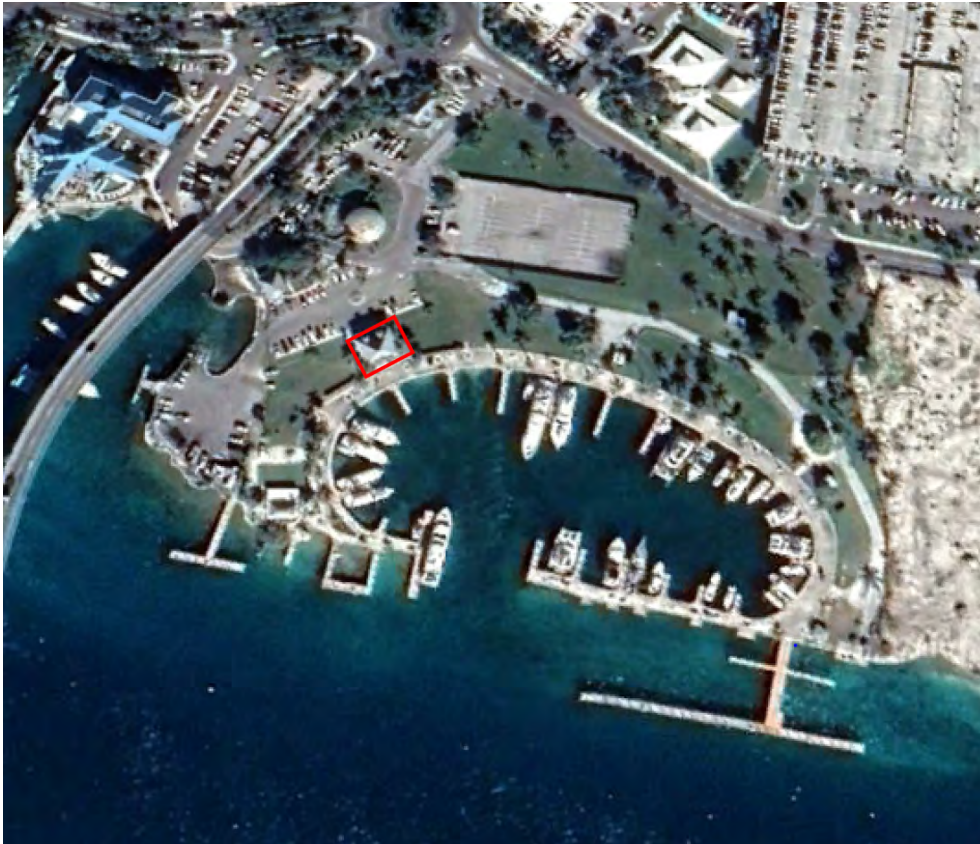
Figure 1: Location of building
