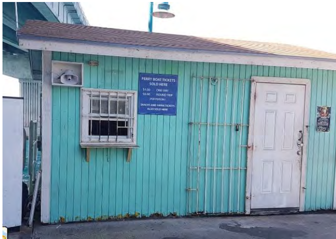
Ferry Terminal Ticket Office Ferry Boat office
