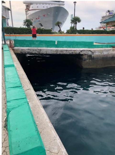
Figure 22. Channel opening to allow water movement at the Tour Boat Operation site.
