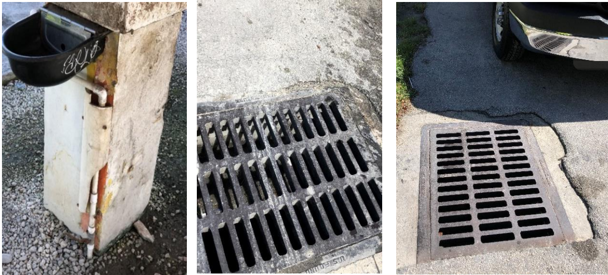
Figure 67. (Left) Potable water connected to horse troughs (Center and Right) Drains within the boundary of the Port.
