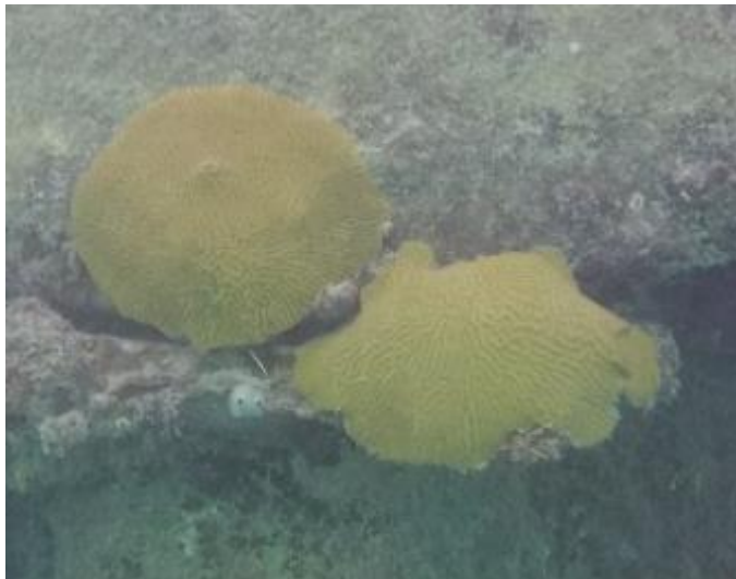
Figure 37. Symmetrical Brain Coral attached to Woodes Rodgers Walk concrete structure.
