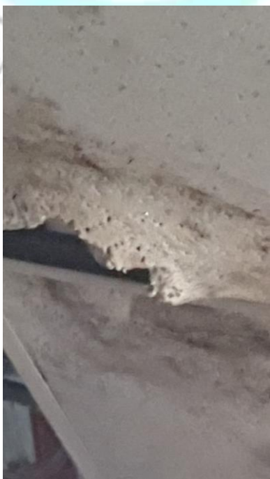
DRYWALL AND TILE CEILING AREAS DAMAGED BY WATER LEAKS
