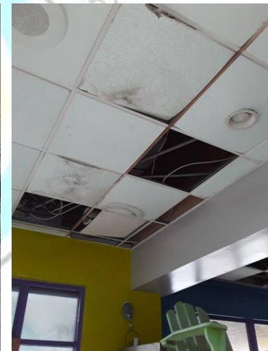
DRYWALL AND TILE CEILING AREAS FOR MOLD REMOVAL
