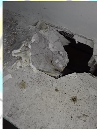
DRYWALL AND TILE CEILING AREAS FOR MOLD REMOVAL
