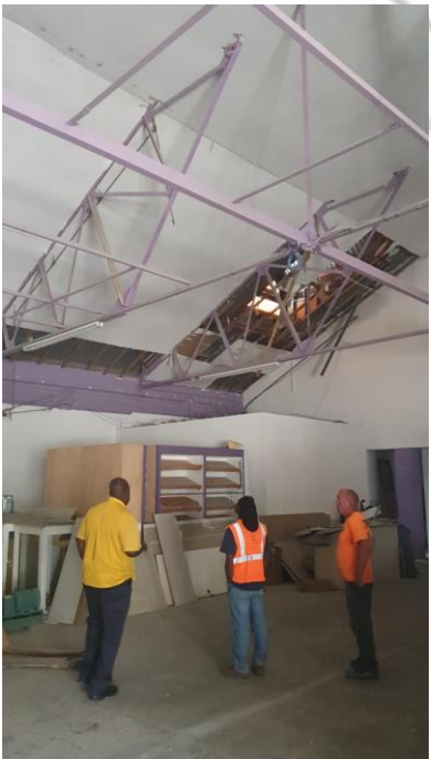
DRYWALL AND TILE CEILING AREAS DAMAGED BY WATER LEAKS
