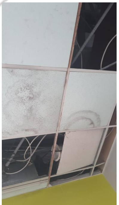
DRYWALL AND TILE CEILING AREAS DAMAGED BY WATER LEAKS
