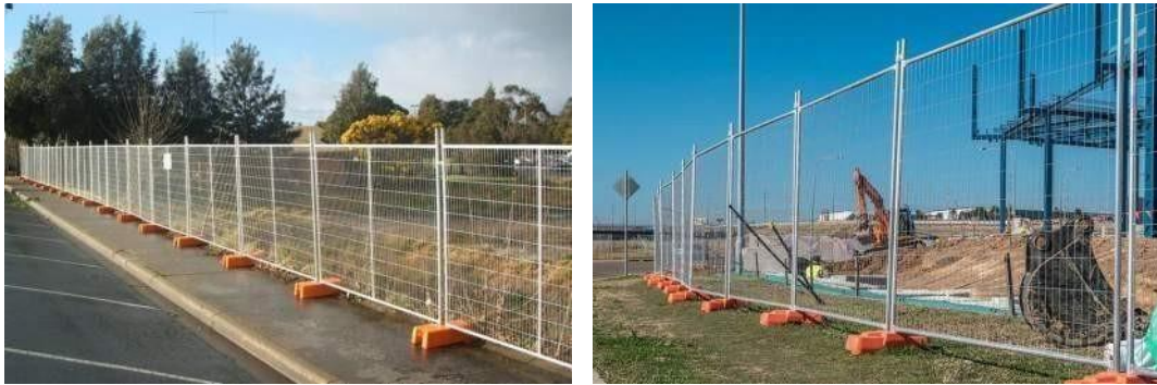
Figure 7. Examples of wired construction fences 3 & 4 .
