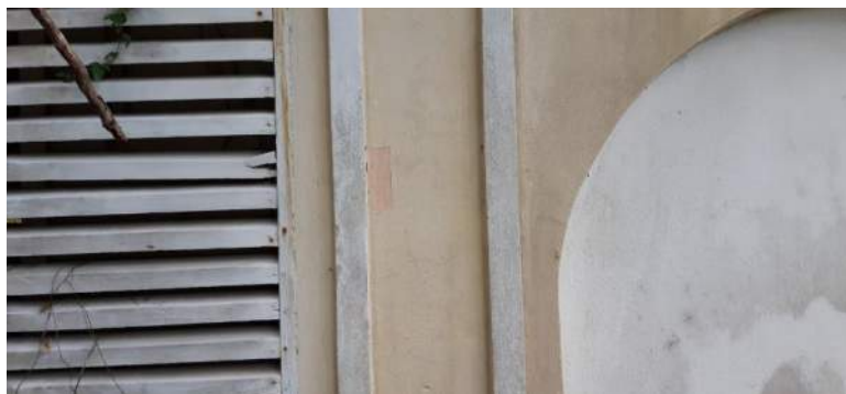
Figure 42. Sample location Pump House, lead sample taken from exterior paint
