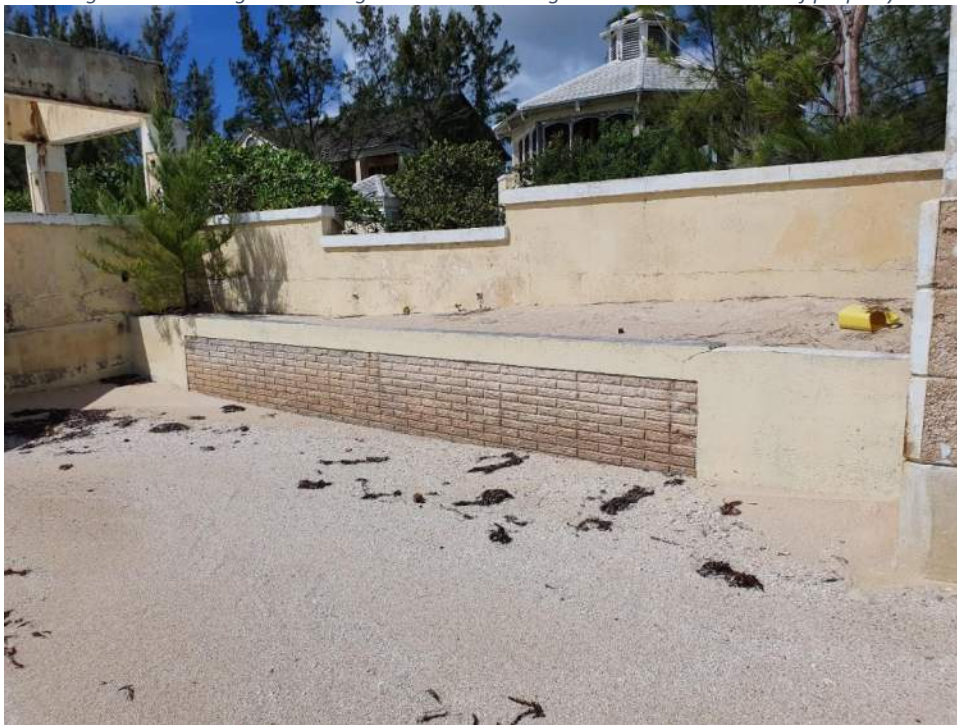
Figure 17. Existing seawall in good condition along the southern shoreline of property
