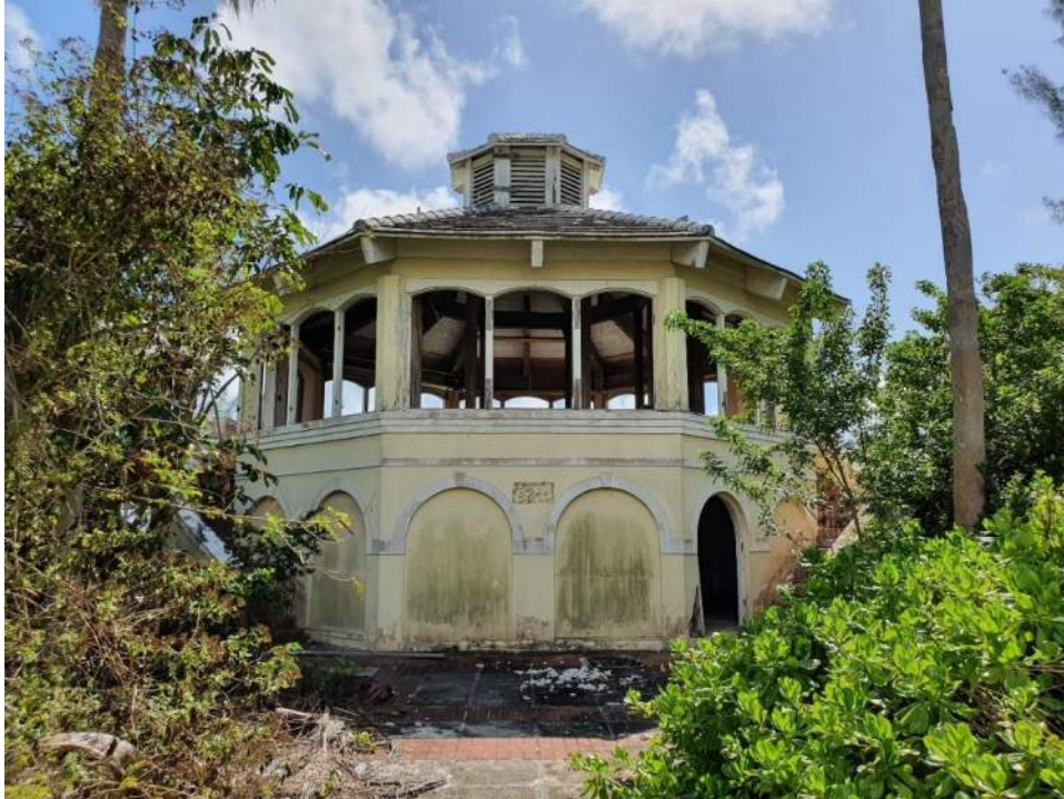
Figure 7. Exterior of pool kitchen at former South Ocean Resort
