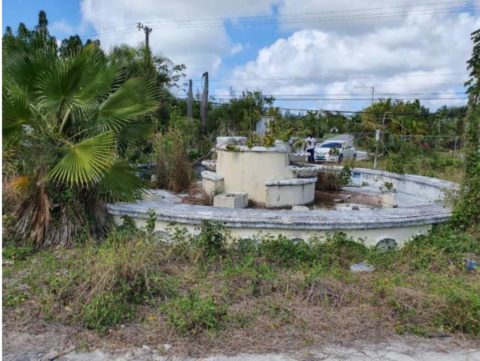
Figure 6. Water fountain within center courtyard at former South Ocean Resort
