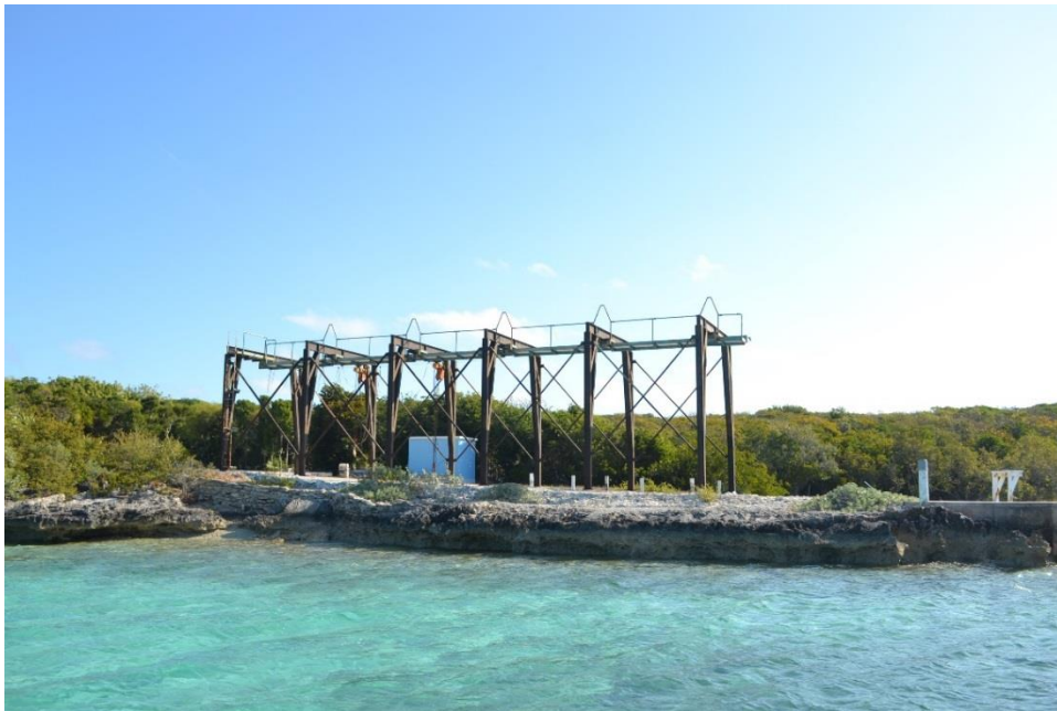
Photo 4-46. WT115: Boat Hoist with Concrete Boat Ramp on Far Side of Hoist
